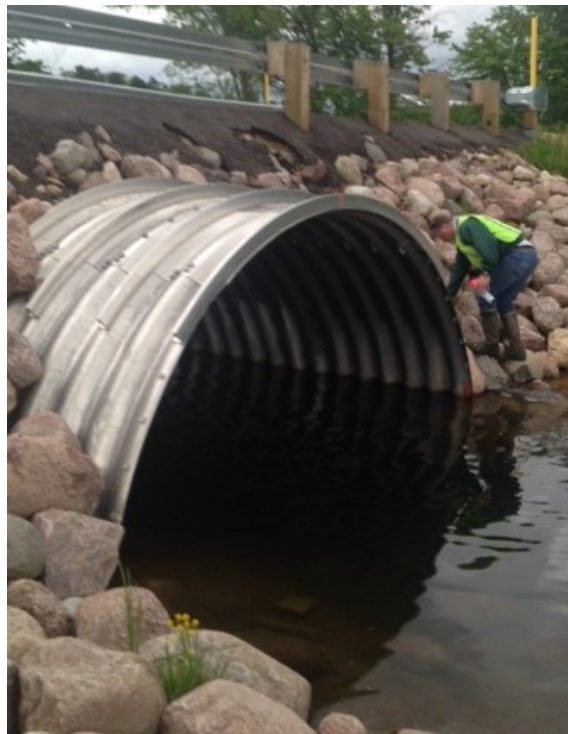
Miles Winkler, left, DNR water management engineer, lines up surveying equipment to reset water level measurements on the new culvert on Highway Y by the boat launch site. Scott Koehnke, right, DNR water management specialist, marks the elevation on the culvert. The culvert has been the official lake level bench mark, which had to be reset after the culvert was replaced last year. Official levels in feet above sea level are: marked bolt: 800.44; high water: 799.88; normal: 799.58; low: 799.28.
